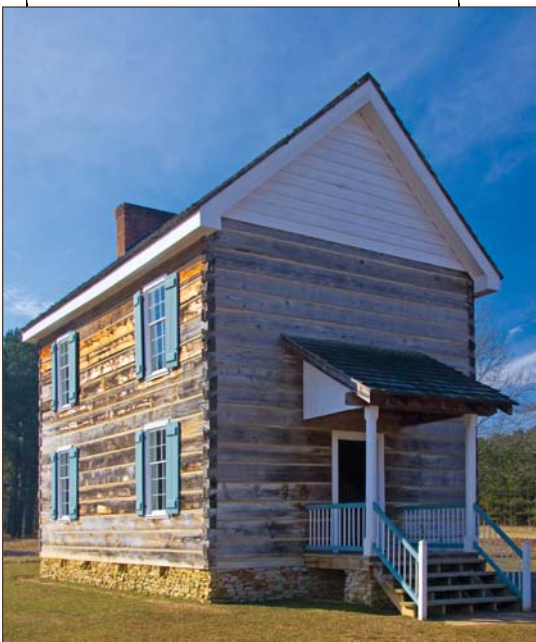
Buildings at New Echota have been reconstructed on its original site, with the Cherokee Phoenix office (top, on the left), Cherokee Supreme Court (top, on the right), and Council House (above).
