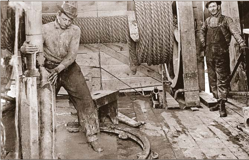
This is the mouth of an 18-inch drilling bit hole on a derrick floor at the Drumright oil field.
