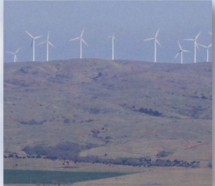
The Blue Canyon wind farm is located near Lawton, OK.
