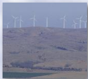
The Blue Canyon wind farm is located near Lawton, OK.
